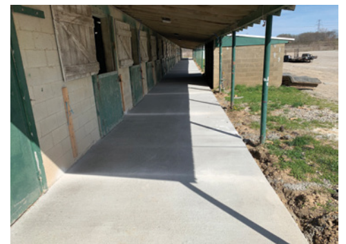
Concrete and gravel have been added to the barn area.
